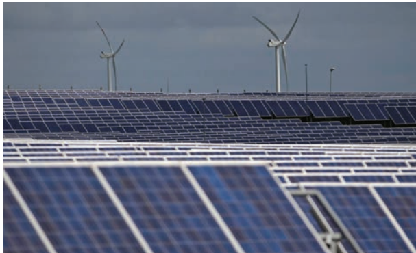
Kamuthi solar power plant
