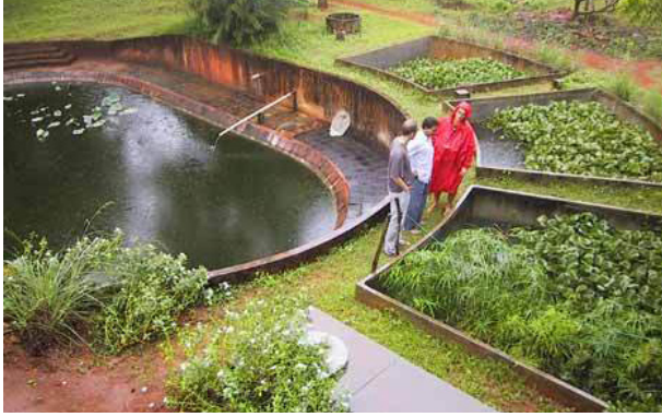
Fig .13.7 (a) DEWATS System at Auroville
